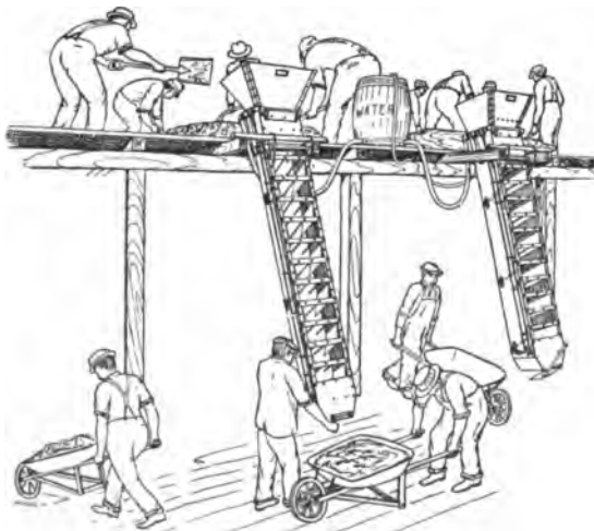
Fig. 35.—The Gravity Concrete Mixer.
